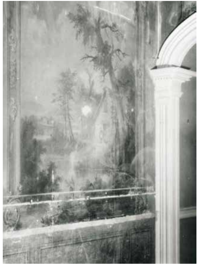
Mural, before restoration, 1931.
