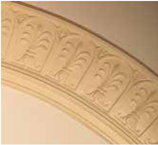
Ceiling, plaster, about 1910.
